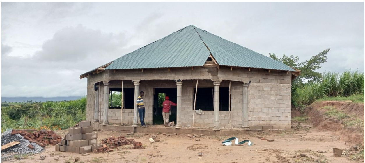
The kitchen construction (at roofing level)
